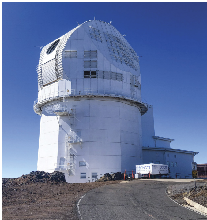
▲ EYE OPEN DKIST stands with open aperture beneath a blue sky near the summit. A series of windows called vent gates enables operators to control the temperature and airflow inside the enclosure, keeping equipment stable in a variety of conditions.
