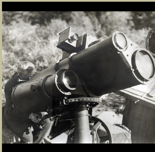
▲ MIGHTY MACHINE Barnard is photographed seated at the Bruce 10-inch photographic telescope on Mount Wilson. In addition to the 10-inch Brashear lens, a 6¼-inch Voigtländer lens, a visual guide telescope, and a smaller camera all shared the same mount.
