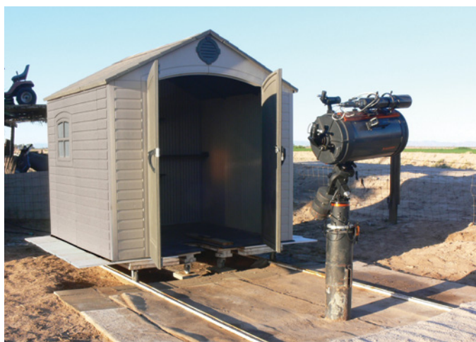
▲ Left: When closed, Laird Stiegler's observatory is just a commercial storage shed on a wheeled platform. Right: The entire building rolls away, leaving the telescope on its pier with a view down to the horizon on three sides.
