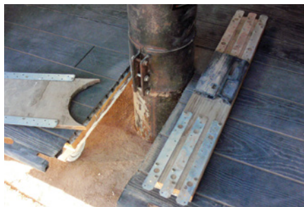
▲ The floor is cut out to accommodate the telescope pier. A removable section seals the slot tight against intrusive creatures. The section to the right is a brace that goes under the sill.
