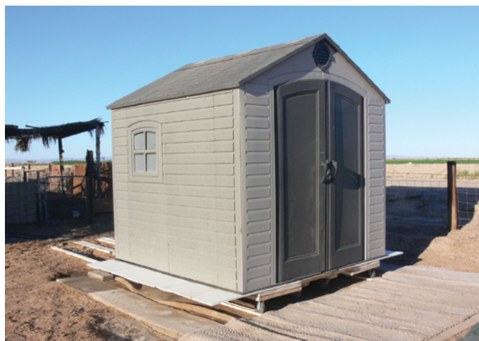
▲ Left: When closed, Laird Stiegler's observatory is just a commercial storage shed on a wheeled platform. Right: The entire building rolls away, leaving the telescope on its pier with a view down to the horizon on three sides.
