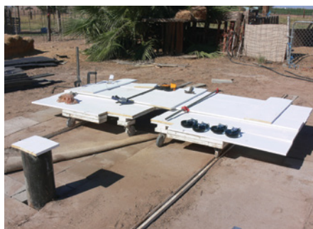
▲ The building rests on a framework of criss-crossed 2" x 10" lumber.
