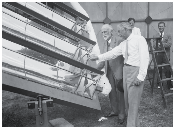
▲ POWERED BY THE SUN Abbot points at one of his solar-powered boilers in this 1936 photo. This was just one of the many solar devices he experimented with throughout his life. Steam generated by this device could power an engine.
