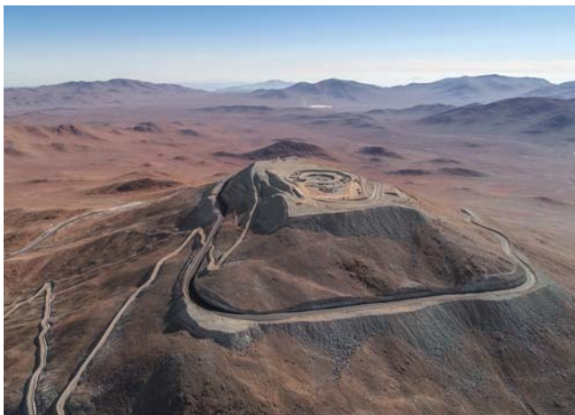
▲ FUTURE ELT SITE Taken in early 2018, this image shows the early foundations for the dome and telescope structure of ESO's Extremely Large Telescope (ELT), which will perch at an altitude of some 2,500 meters (8,300 feet) on Cerro Armazones in the Chilean Atacama Desert.
