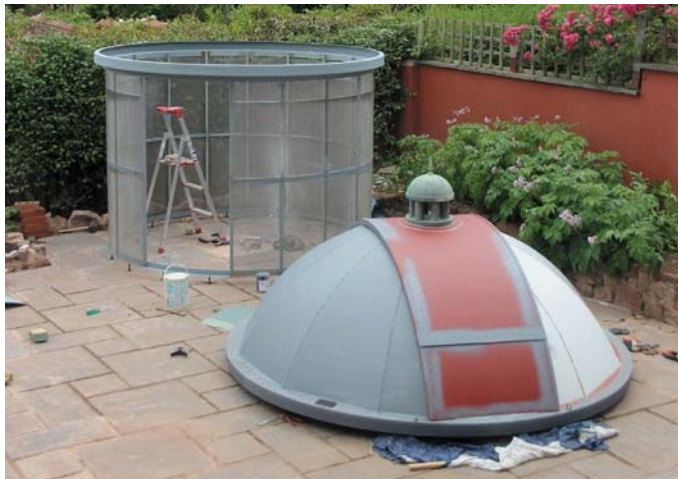
▲ STEEL SKELETON The walls of the observatory were constructed of welded galvanized steel surrounded by perforated mesh used to secure the adhesive to affix the brick facade.
