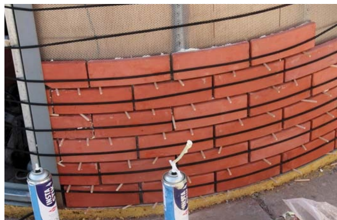
▲ BRICK MOLD To reduce thermal issues from traditional bricks, the author fabricated custom "bricks" from a concrete and fiberglass mixture in a custom mold designed to match the radius of the walls. Right: Each brick was then mounted using a foam adhesive and strapped into place using bungee lines while the adhesive set. The final structure is 2½ meters (8.2 feet) in diameter by 3 meters tall, with a 60-centimeter-wide (24-inch) slit.
