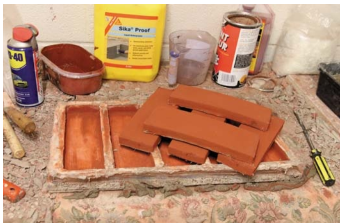
▲ BRICK MOLD To reduce thermal issues from traditional bricks, the author fabricated custom "bricks" from a concrete and fiberglass mixture in a custom mold designed to match the radius of the walls. Right: Each brick was then mounted using a foam adhesive and strapped into place using bungee lines while the adhesive set. The final structure is 2½ meters (8.2 feet) in diameter by 3 meters tall, with a 60-centimeter-wide (24-inch) slit.
