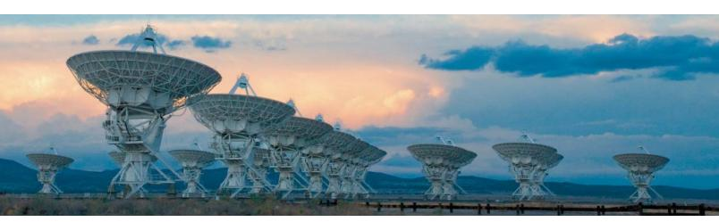
▲ **THE LISTENERS** The Karl G. Jansky Very Large Array in Socorro, New Mexico, consists of 27 radio dishes each 25 meters (82 feet) in diameter. Their data are combined interferometrically to create radio images with the sensitivity of a single 130-m dish, but with much higher spatial resolution.
