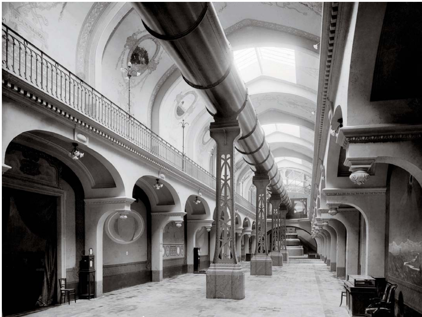
LIGHT PIPE Two hundred feet of steel pipe, weighing more than 10 tons, encircled the light beam on its way to focus. A cloth shroud or even just a few light baffles might have done better; telescope makers have learned to keep as much mass as possible away from the light path to reduce distorting thermal effects. Observers thought that the city air was causing poor images, but the massive, unventilated metal tube could not have helped.
