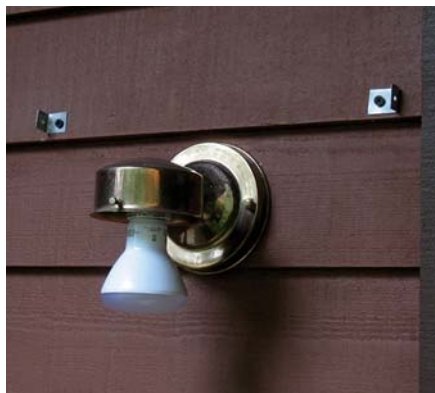
▲ Left: Replace the carriage light with a downward-facing fixture and a downward-facing flood bulb. Note the brackets for mounting the shield that are attached to the siding. Middle: Install the brackets on the wall, and then attach the shield (shown assembled). Right: The finished shielded fixture casts its light downward where it's useful, not outward into your eyepiece.
