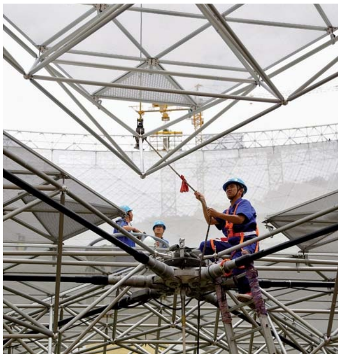
▲ JIGSAW PUZZLE On July 3, 2016, workers installed the last of 4,450 triangular panels that form the telescope’s reflective surface.
